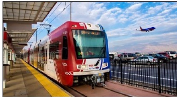
LIGHT RAIL – OKC-WILL ROGERS AIRPORT
